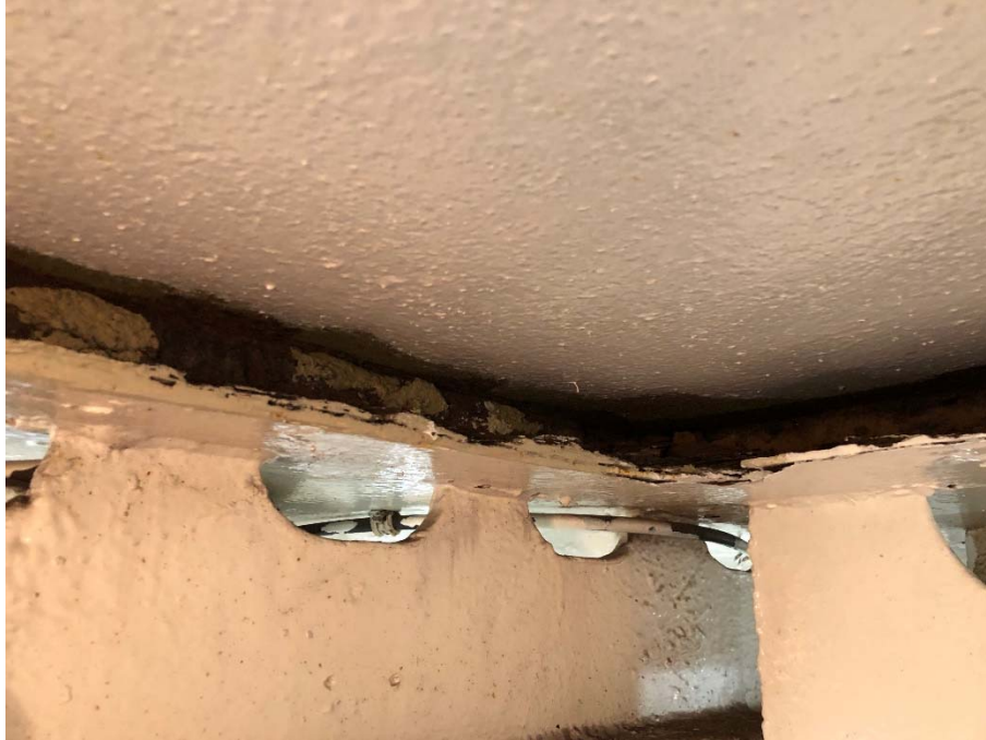
Figure 8 - Top deck plating seen through opening in original deck plating
