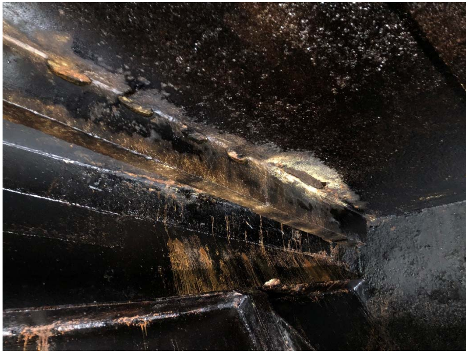
Figure 6 - Typical state of original deck plating in FWD void space
