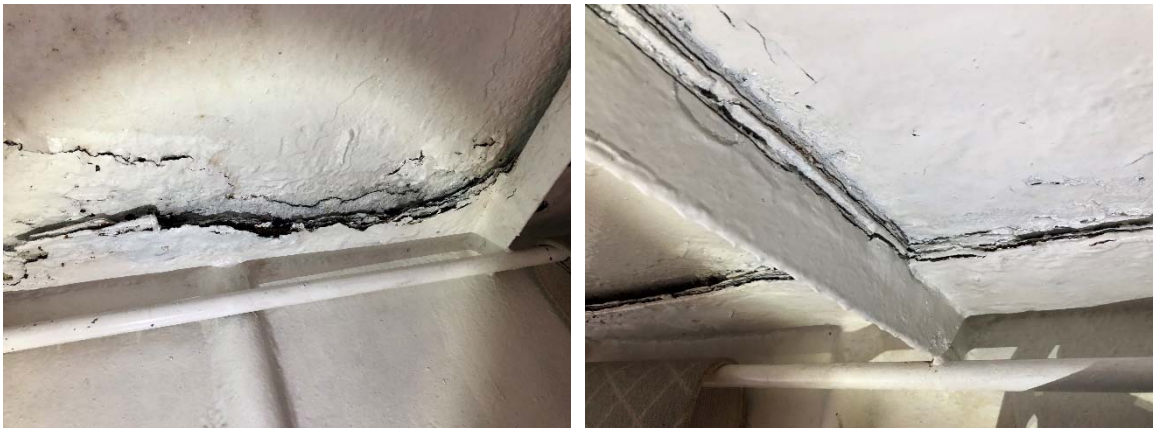
Figure 22 – Plating of deckhouse, seen from below
