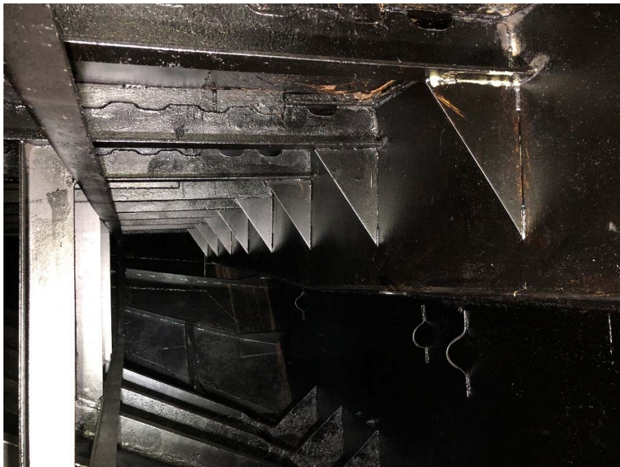
Figure 15 - Stiffeners and flatbars in Aft void space
