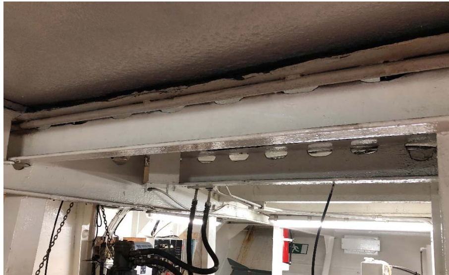
Figure 12 - Typical condition of a deck longitudinal
