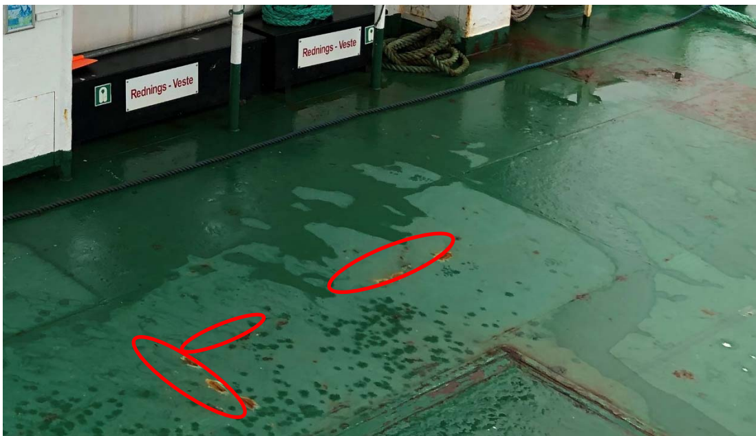
Figure 2 - Slot welds, visible from above deck
