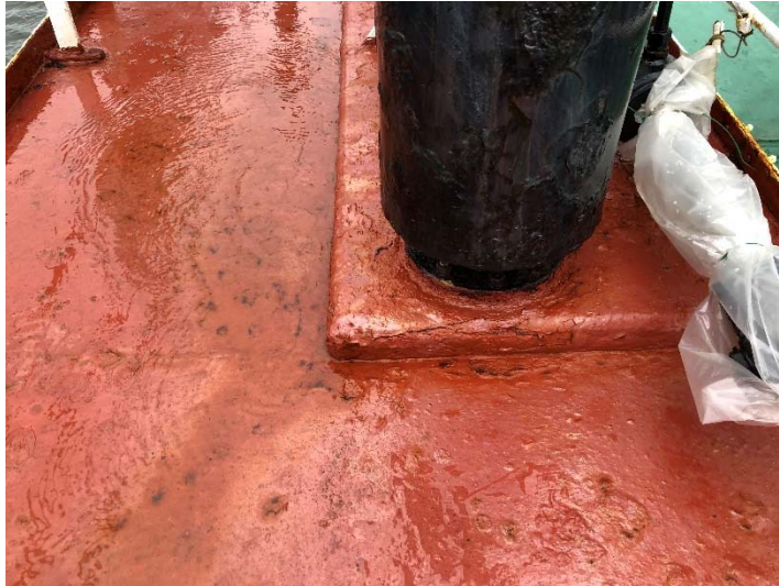
Figure 23 - Plating from deckhouse, seen from above
