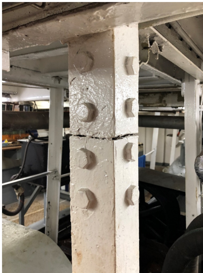
Figure 19 - Pillar bolted connection
