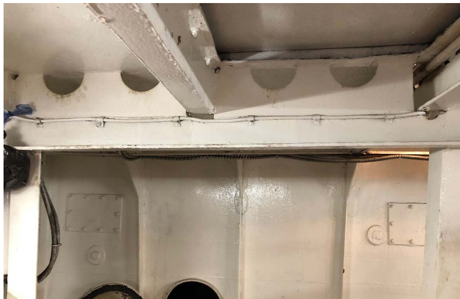
Figure 13 - Typical condition of a web frame
