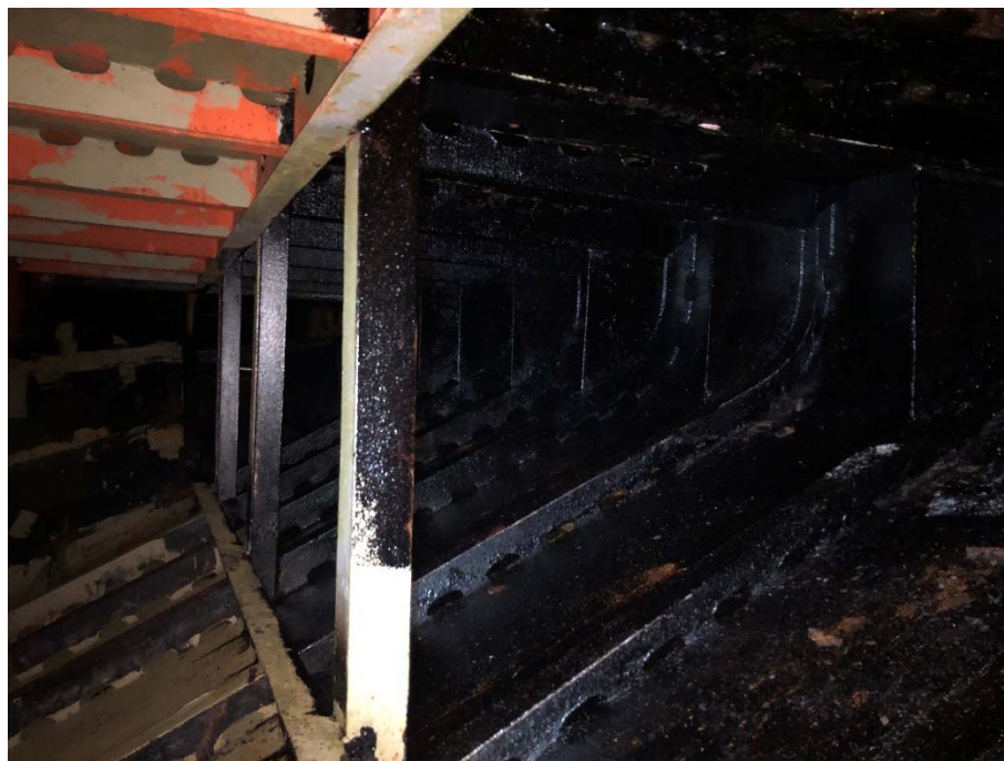
Figure 17 – Stiffeners and original deck plating in Fwd void space
