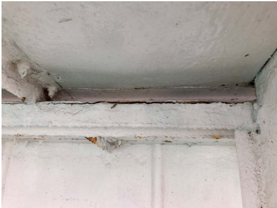
Figure 26 - Cover plate under passenger platform planking
